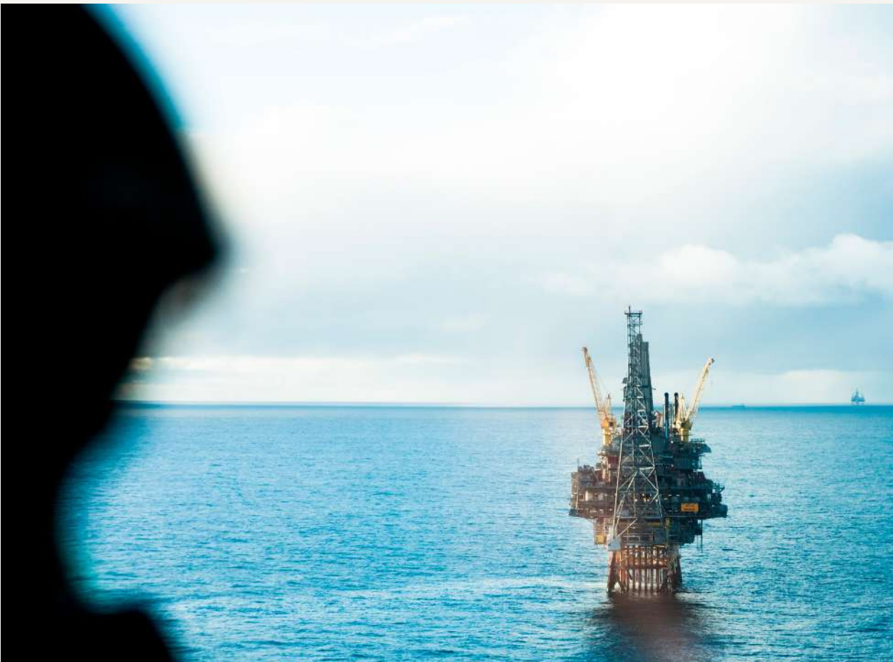
The Brage Platform while approaching it with a helicopter. Credit: OKEA ASA
